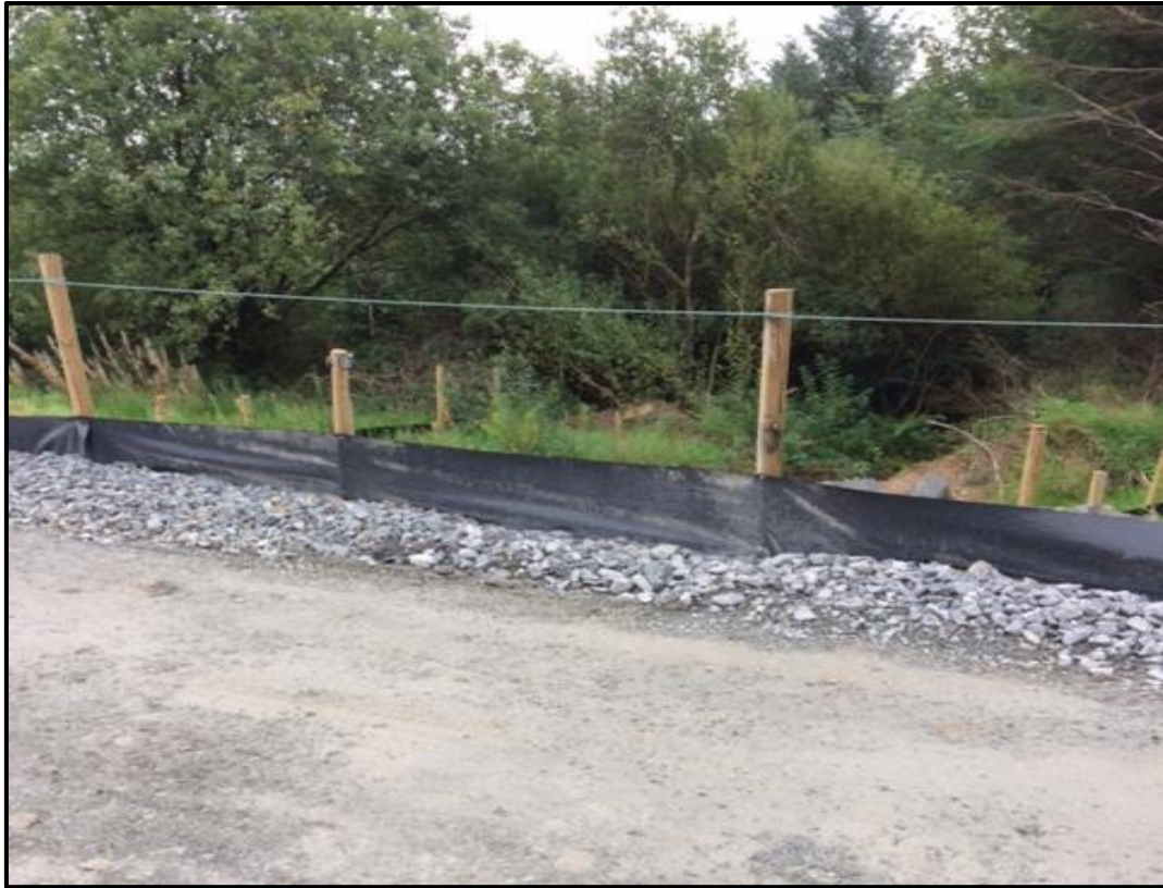
Figure 3-17: Dirty water containment at watercourse crossings
