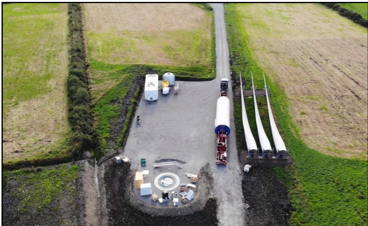
Figure 3-6: Typical finished hardstand on a wind farm
