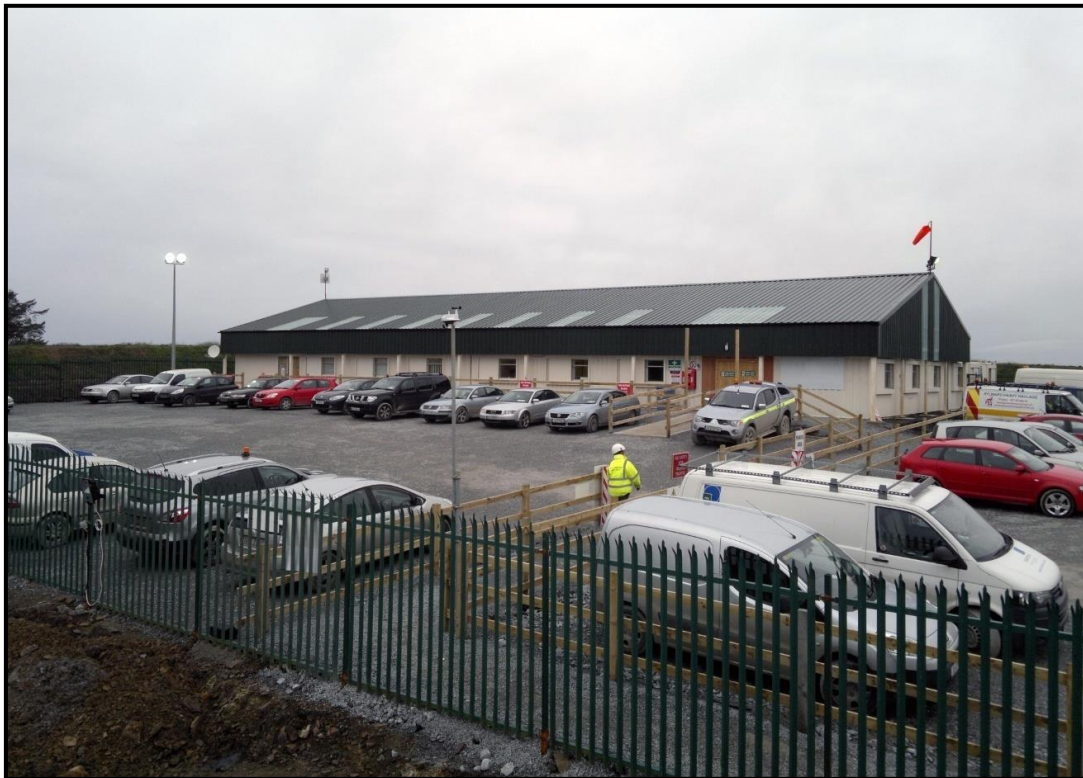
Figure 3-12: Typical temporary site construction compound on a wind farm
