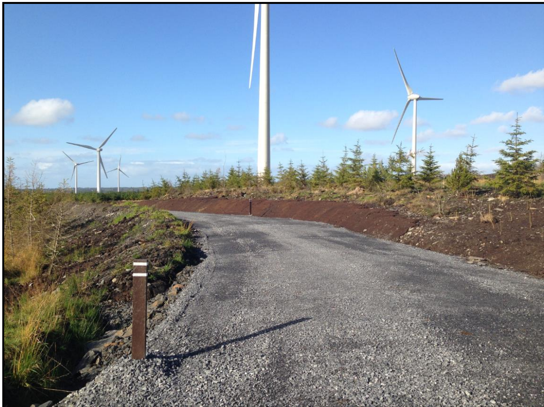
Figure 3-4: Typical new excavated access track on a wind farm
