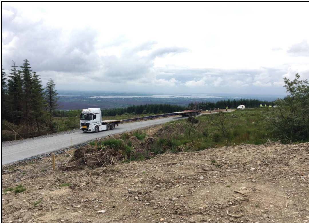
Figure 3-3: Typical upgraded track on a wind farm
