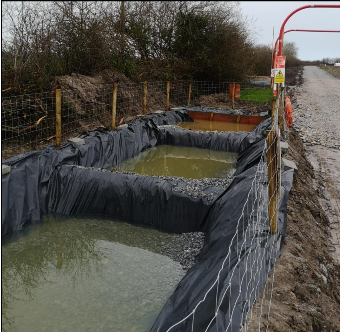
Figure 3-20: Multi-tiered settlement pond with stone filter
