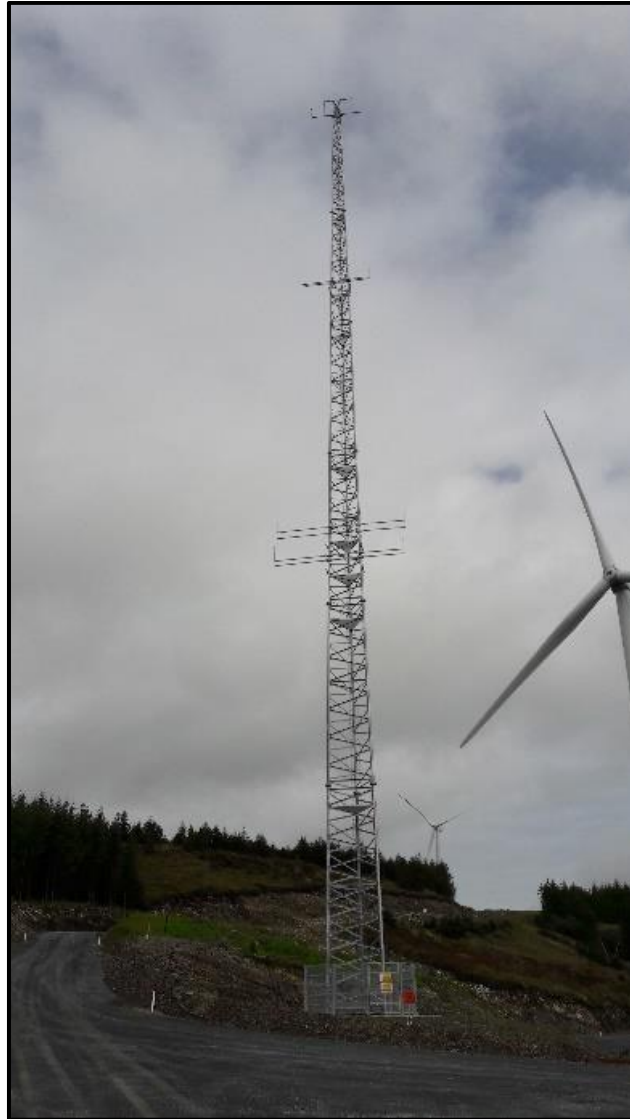
Figure 3-11: Typical meteorological mast on a wind farm
