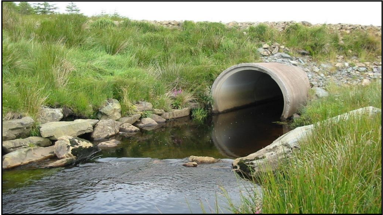
Figure 3-16: Typical concrete pipe channel crossing
