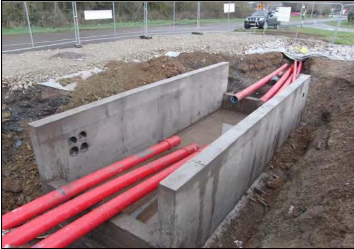
Figure 3-9: Typical joint bay construction
