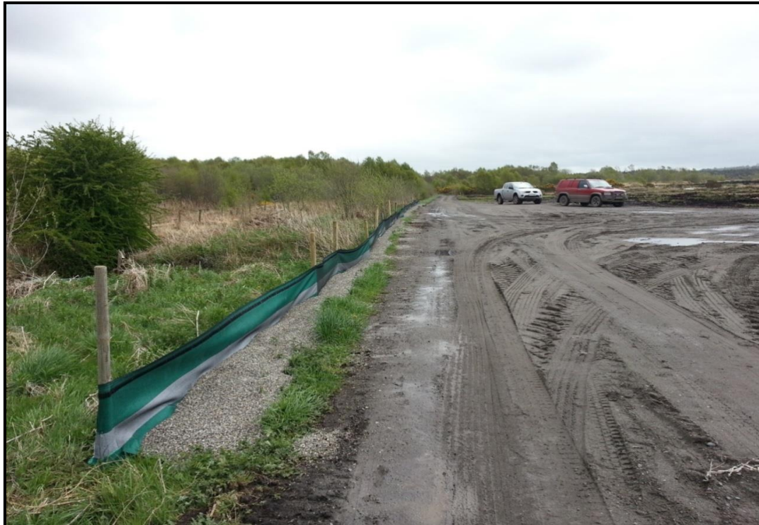
Figure 3-18: Silt curtain containment along tracks near watercourses
