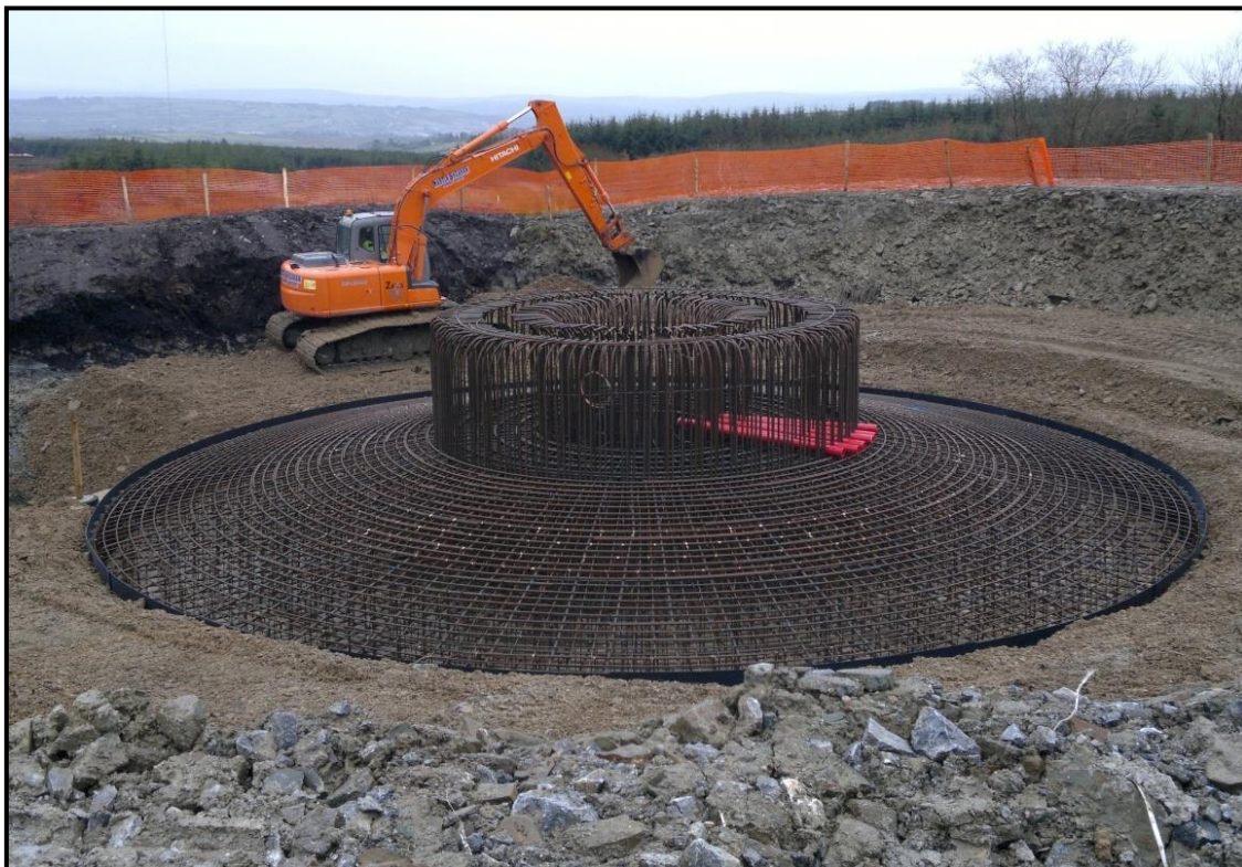
Figure 3-7: Typical construction of a wind turbine base
