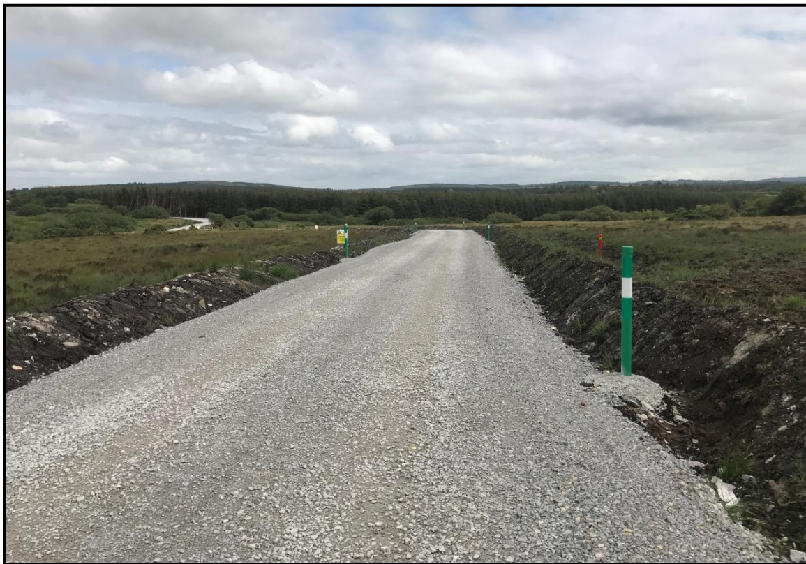
Figure 3-5: Typical floated track on a wind farm
